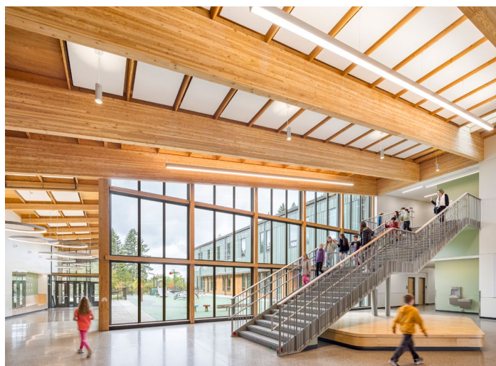
ABOVE Glulams at Art Rutkin Elementary School (Photo credit: Josh Partee)
