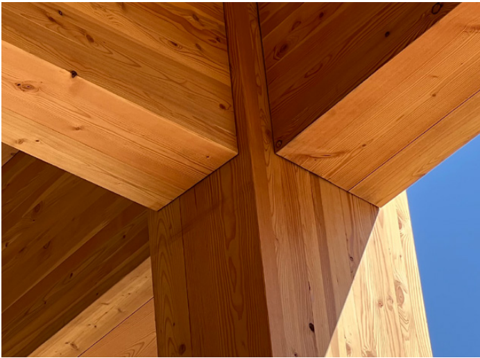
ABOVE Small gaps are anticipated between structural members, like between these beams and column.
